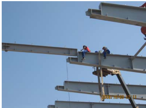
a. King post rafter positioning
