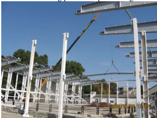
a. King post rafter positioning
