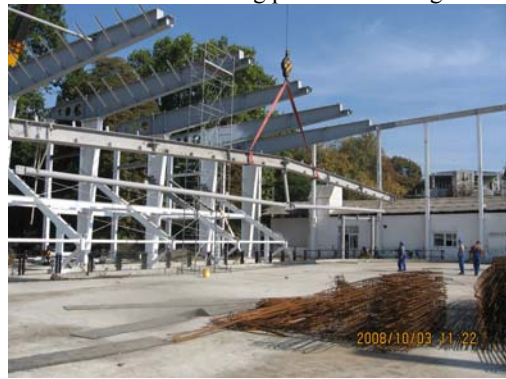
b. King post rafter lifting
