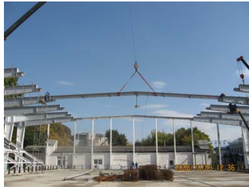
b. King post rafter lifting
