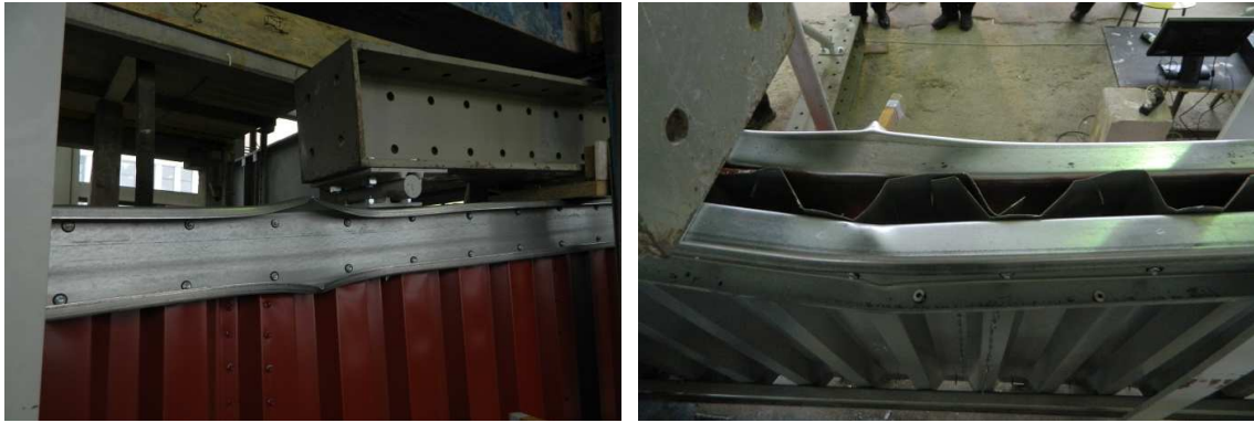
Fig. 10: Failure mechanism on the top flange of Beam-2
